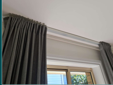
Heavy drapes installed so there is minimal air gap with the ceiling
